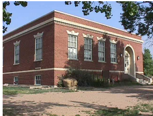
Building in Lamar
